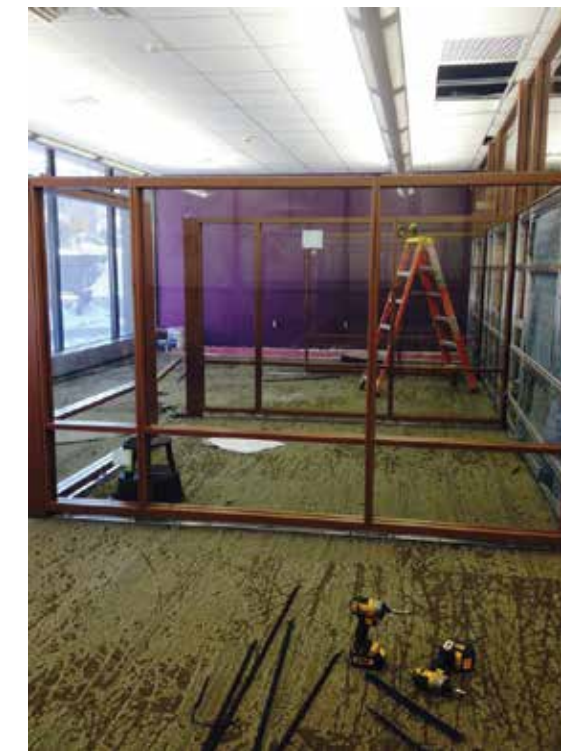
The BioCommons under renovation during winter break, 2014-15.
